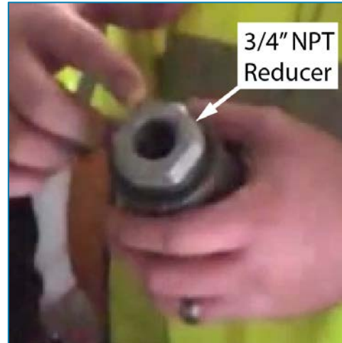
Figure 2-2 Flange with 3/4-inch Reducer
