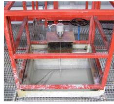
In the site of the tank park rainwater is collected to underground tanks. Rainwater tanks are instrumented with NIVELCO NIVOSWITCH RCM-400-3 vibration fork level switches. Emptying of the rainwater tanks are performed by hand-intervention based on the signals of the level switches.
