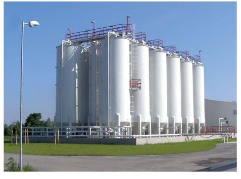
The outside tank-park contains different quality, density, or diverse doped mud. Level transmitters and switches
