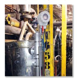
display. The bypass chamber is equipped with a NIVOTRACK magnetostrictive level transmitter which performs high accuracy level measurement and displays the level on the SAP-300
