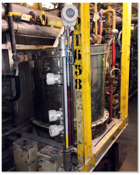
plug-in display module and transmits the measurement data to the central control room. The bypass chamber is also equipped with 3 MAK-100 level switches performing high limit, low limit, and low fail-safe level alarm indications. The temperature of the stored demineralised water is 80 °C (176 °F) and the process pressure is atmospheric. The next step of the manufacturing process after cleaning is the heat treatment.
