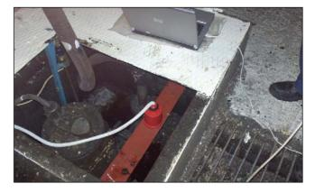
In case of high fail safe indication, the transmitter records the last true measured value and keeps the pump working. The pumps of the full tanks start emptying when authorized by the level transmitter of the separator tank. When the programmed low level is reached, the level transmitter stops
