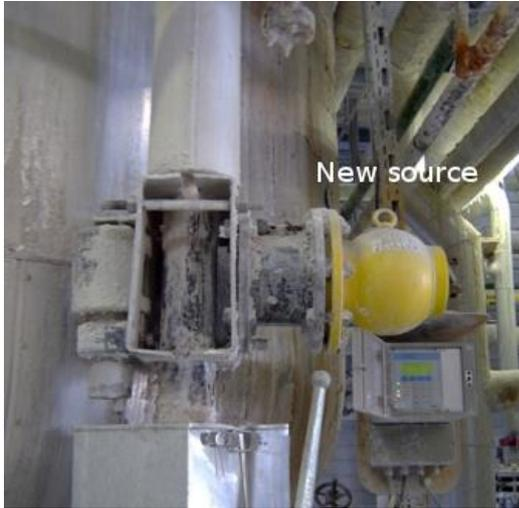
The shielding of some of the old nuclear density meter installations are in terrible shape which means that it is not safe for employees to work with these devices. Staff can be exposed to the radiation without health risks for a short time. However, it is unhealthy when the staff is working around these (old) nuclear devices for longer periods of time.
