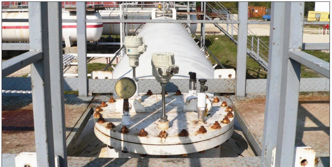
For high alarm indication vibrating forks have been installed.
